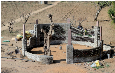
The Pushkar Project: one week into construction, using recycled bricks, glass bottles and reclaimed waste.
